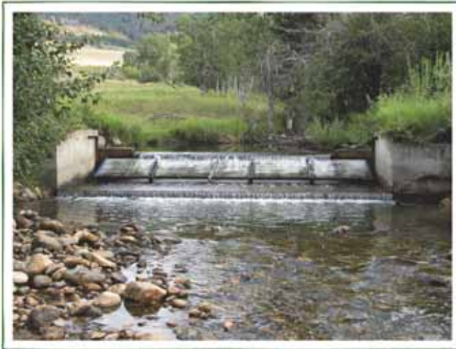
Temporary fish movement barrier on Cherry Creek
