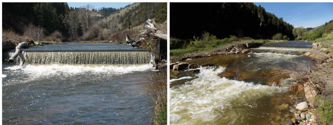
Figure 4. Pre (left) and post (right) photos of Phase-3 barrier showing the results of step pool construction.
