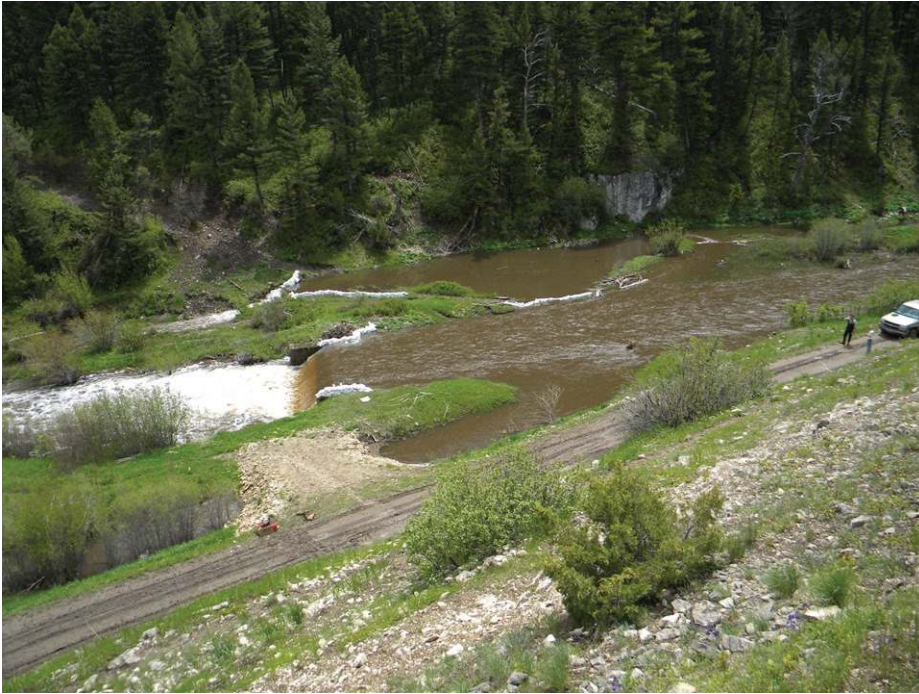
Figure 9. Phase-3 barrier after peak discharge receded and sandbagging was completed to prevent further flooding that potentially could allow fish to pass the barrier.
