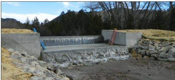
Figure 21: Permanent fish movement barrier on Greenhorn Creek.
