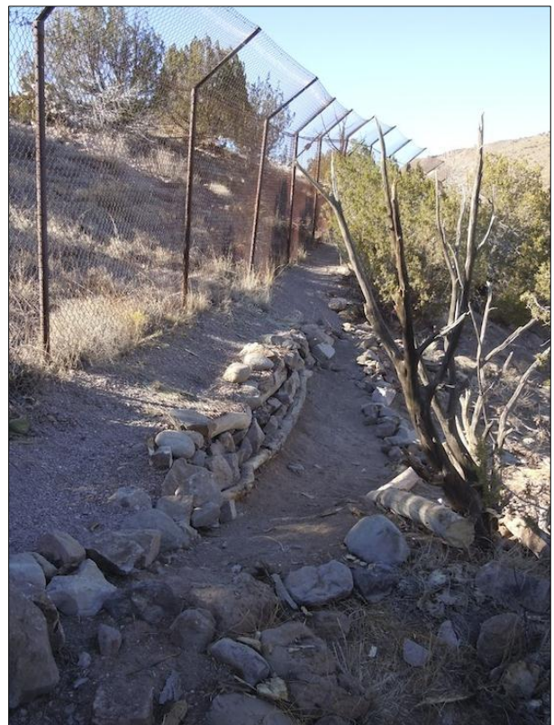
Figure 33: An example of erosion control measures: rock walls, reinforced with logs.
