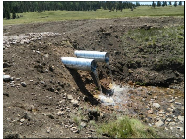
Figure 18: Temporary fish movement barrier on Allen Creek in the Rio Costilla watershed to prevent nonnative fish migration back into a renovated section of the stream.
