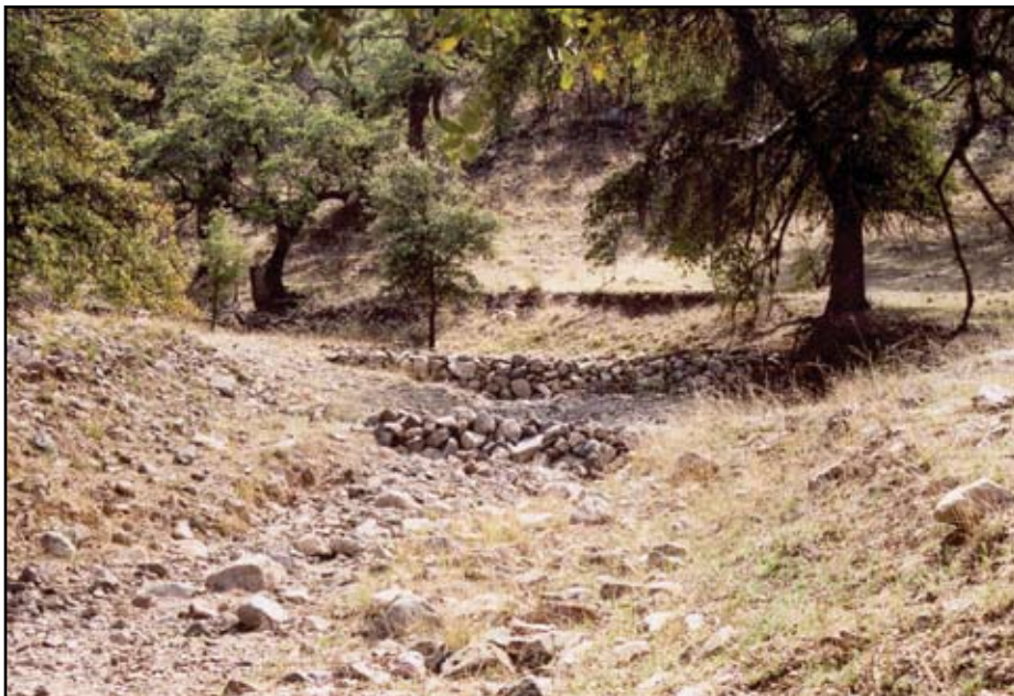
Figure 1. Trincheras (rock curtains), built during spring 2003 retain sediments and increase humidity in Milpillas, Sonora.
