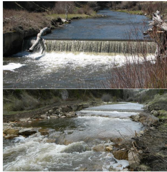
Fig. 12.2. The Cowboy Canyon irrigation diversion (top panel) prevented fish movement from the Butler Section (Phase IV) of Cherry Creek into upper portions of the project area. Installation of rock jump pools now allows fish movement over the irrigation diversion, providing important genetic exchange with the upper watershed.
