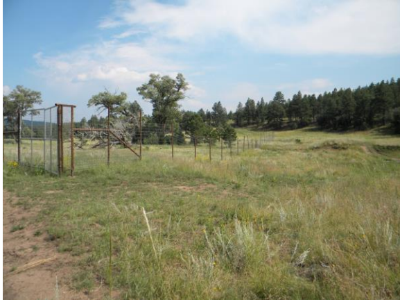
Fig. 12.6. One of ten high fence enclosures to be installed along the upper Vermejo River to improve riparian health.
