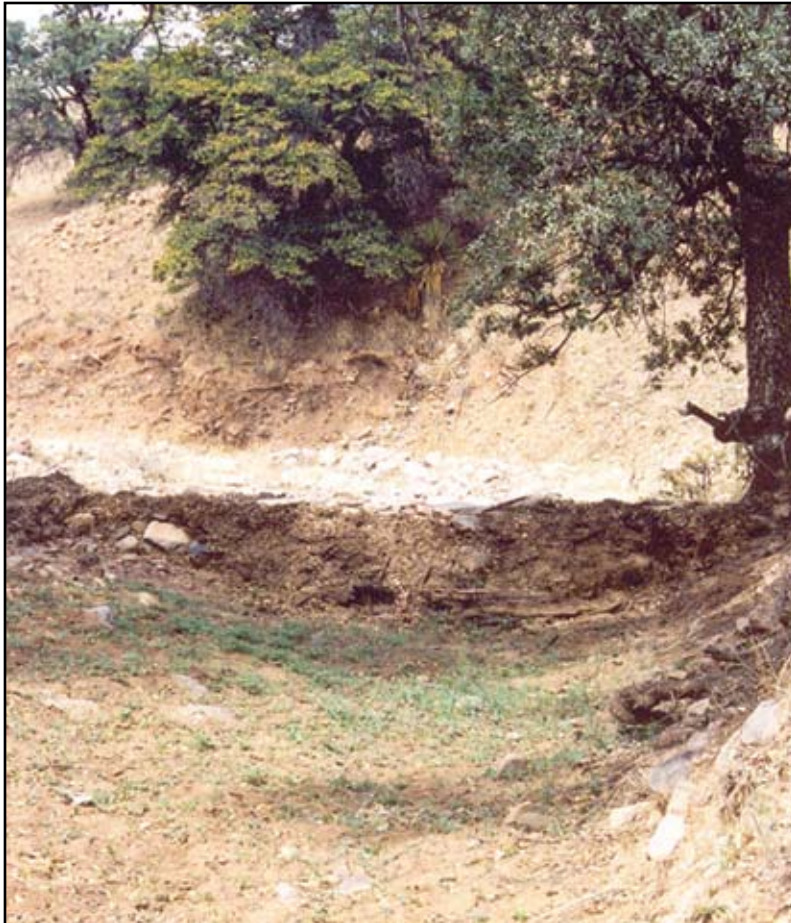
Figure 2. Same trincheras (rock curtains), after summer rains of 2003, showing positive results in soil retention and humidity increment; note new seedlings coming up. Photo by Murrieta and R. Emanuel, 2003.
