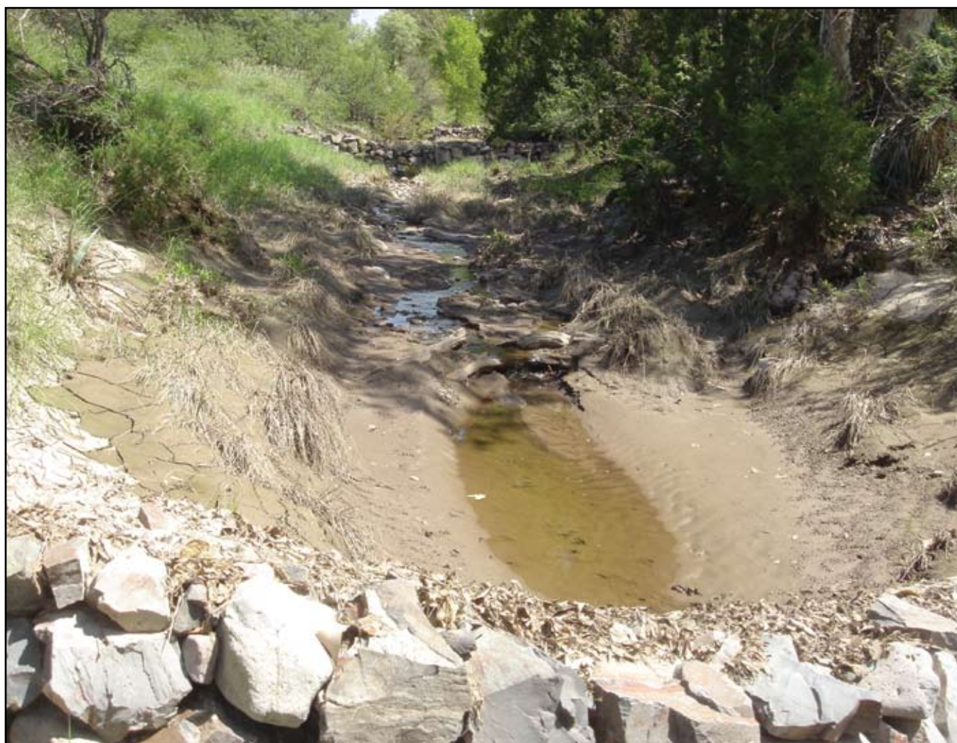
Loose rock structures constructed across streambed.
