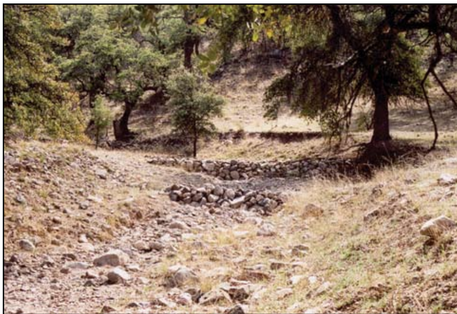
Figure 1. Trincheras (rock curtains), built during spring 2003 retain sediments and increase humidity in Milpillas, Sonora.
