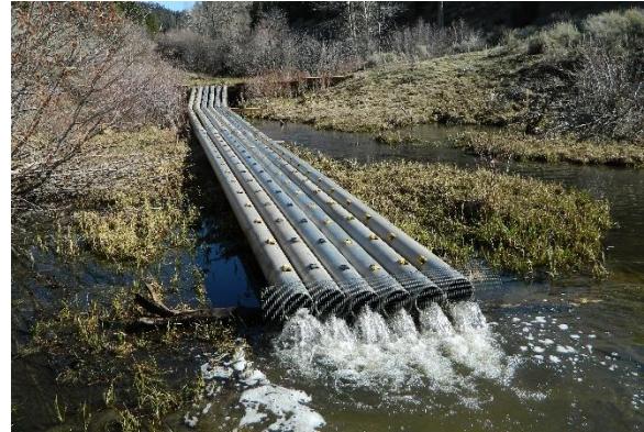
Fig.11.2. Bypass pipes installed at Green Hollow Creek inlet to prevent grayling from spawning in 2016. Note barrier (Fig. 11.1) in background.
