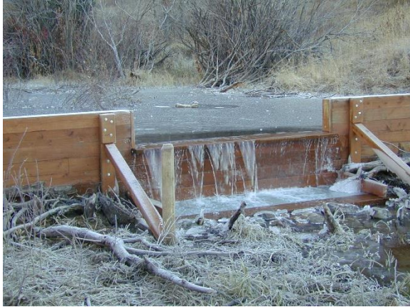
Fig. 11.1. Newly constructed fish movement barrier on Green Hollow Creek in fall 2002.
