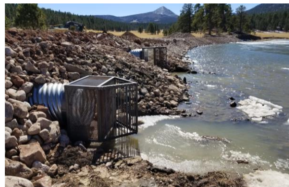
Fig. 10.3. Newly installed fish screens on Munn Lake outlet.
