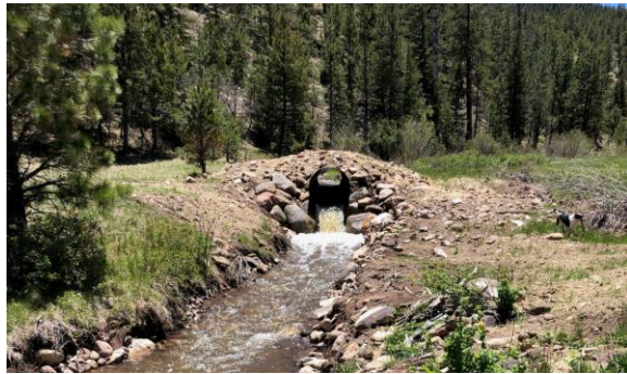
Fig. 10.4. Culvert barrier on Leandro Creek.
