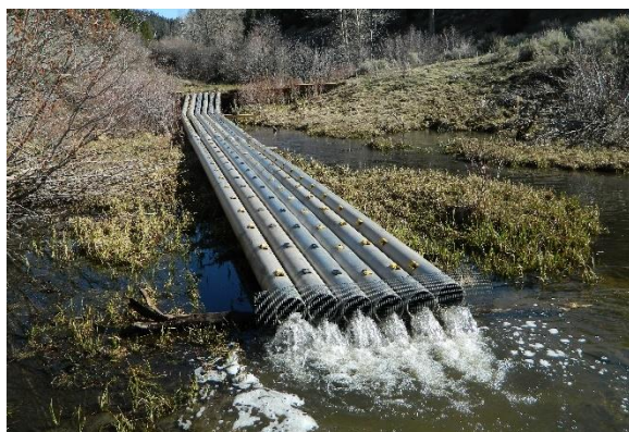
Fig. 11.1. Bypass pipes installed at Green Hollow Creek inlet to prevent grayling from spawning in 2016. Note barrier in background.
